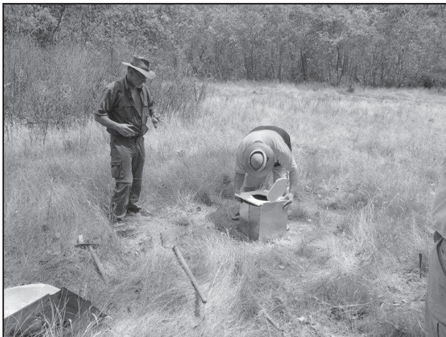
Installing the new flushing toilet at Talooge?
